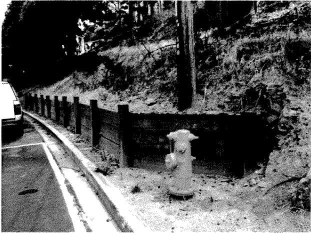
Slope Repair vicinity 266 Santa Clara Street
