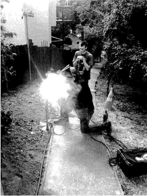
Community Center Handrail
